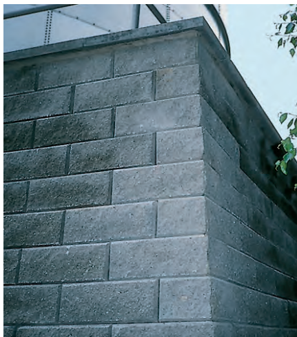
External corner blocks and copings allow neat detailing.
