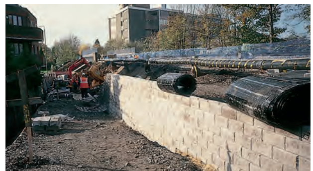
TensarTech TW1 System requires no temporary propping or crane lifts.
