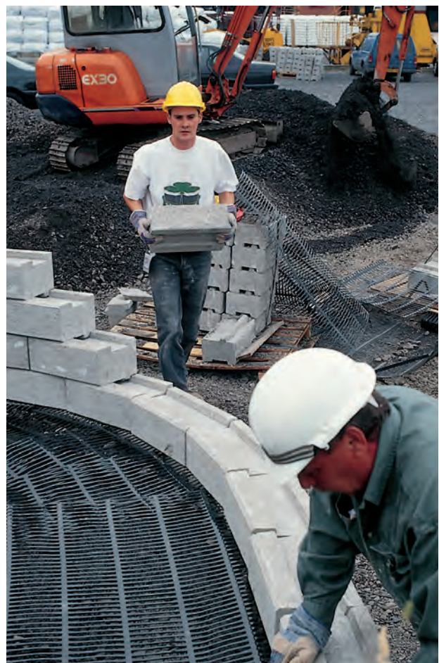
TW1 blocks are delivered on pallets to the point of installation and can easily accommodate tight concave or convex horizontal curves.
