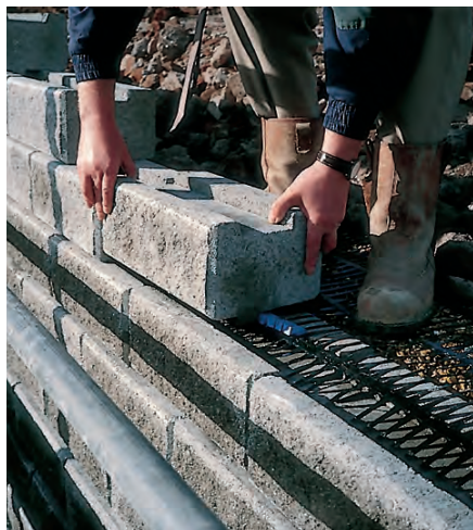
TensorTech TW1 concrete blocks are dry laid, without mortar.
