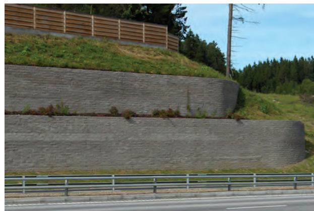
Construction of attractive highways structures with a 120 year design life.
