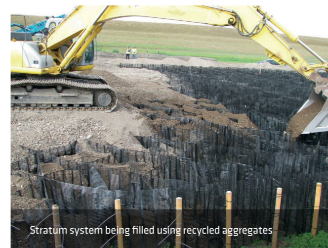
A Stratum system being constructed, Netherlands
