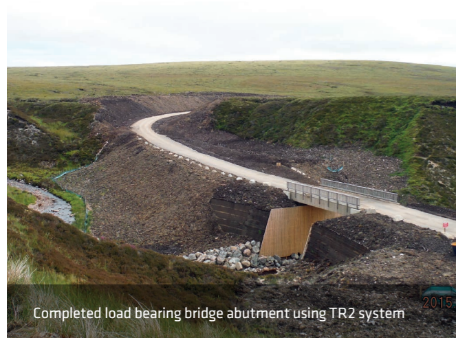
TR2 can be built quickly and easily, without specialist equipment
