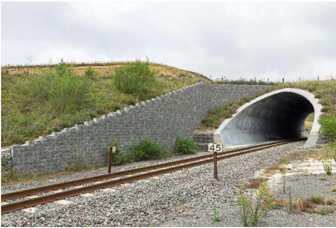
Figure 11. Keystone TW3 western wall in early 2018
