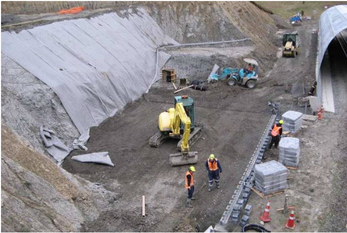
Figure 5. Keystone TW3 east wall at Dashwood at early stage
