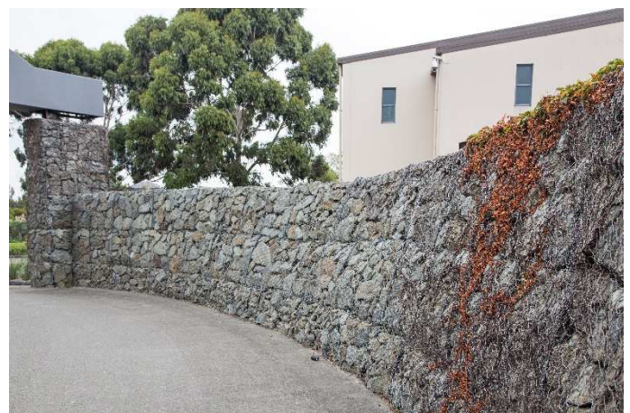
Figure 10. Gabion wall at winery south of Blenheim
