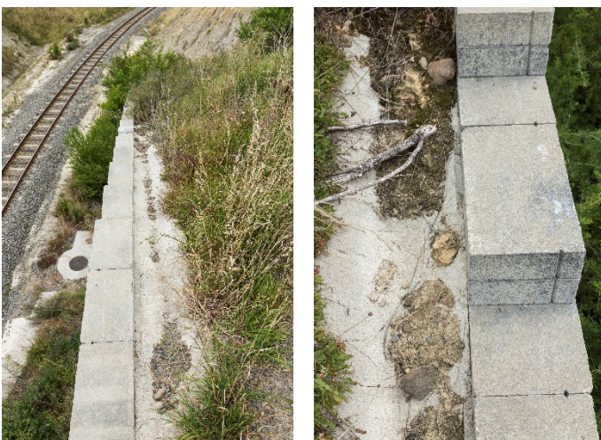
Figure 12. Views of swale drains
