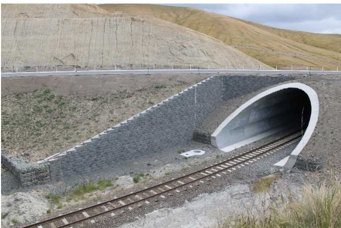
Figure 6. Keystone TW3 west wall at Dashwood completed
