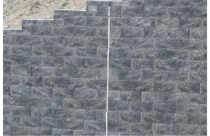
Figure 13. Slip joint pre-earthquake
