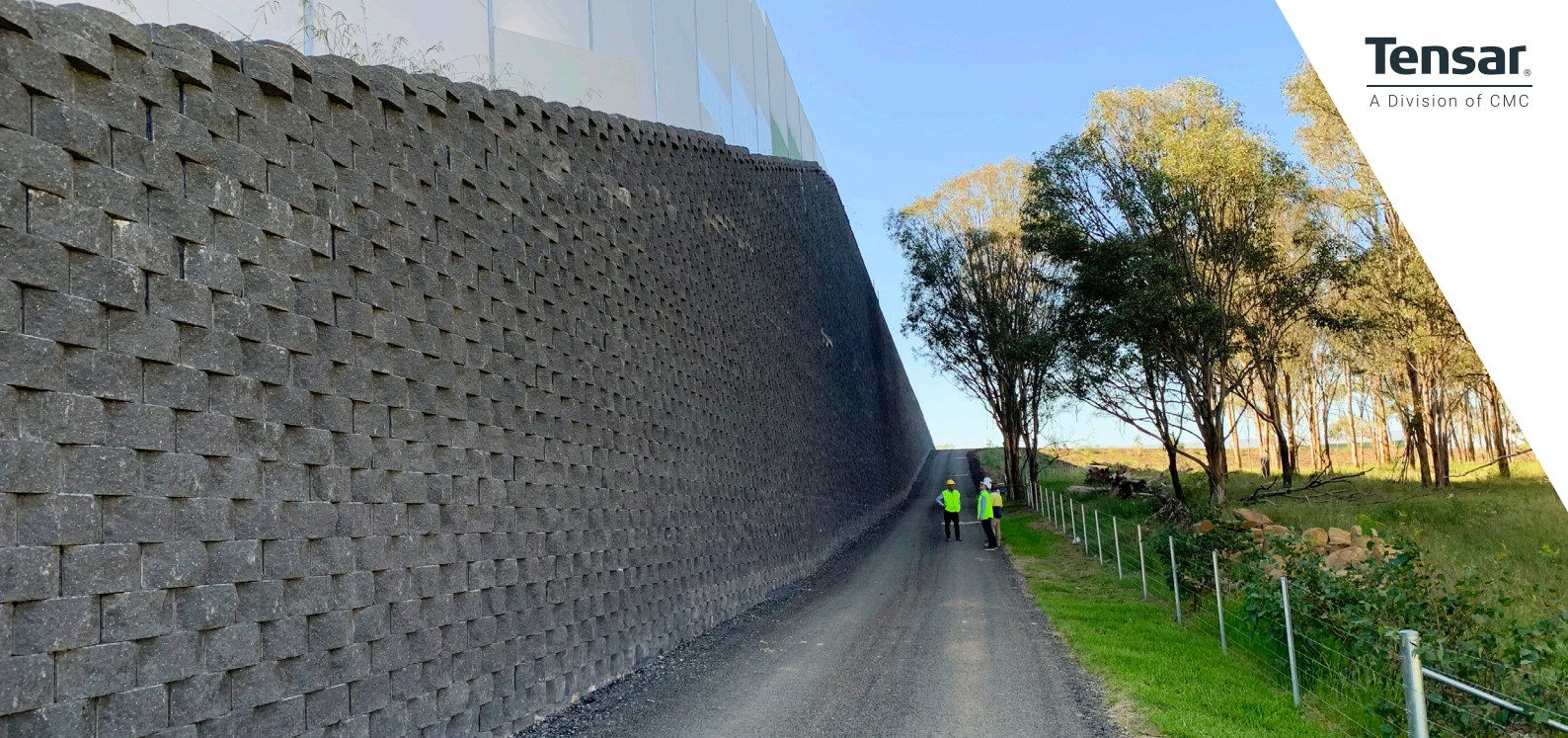
Completed photo of the TensorTech® TW3 Keystone faced reinforced soil retaining wall system in late 2020.
